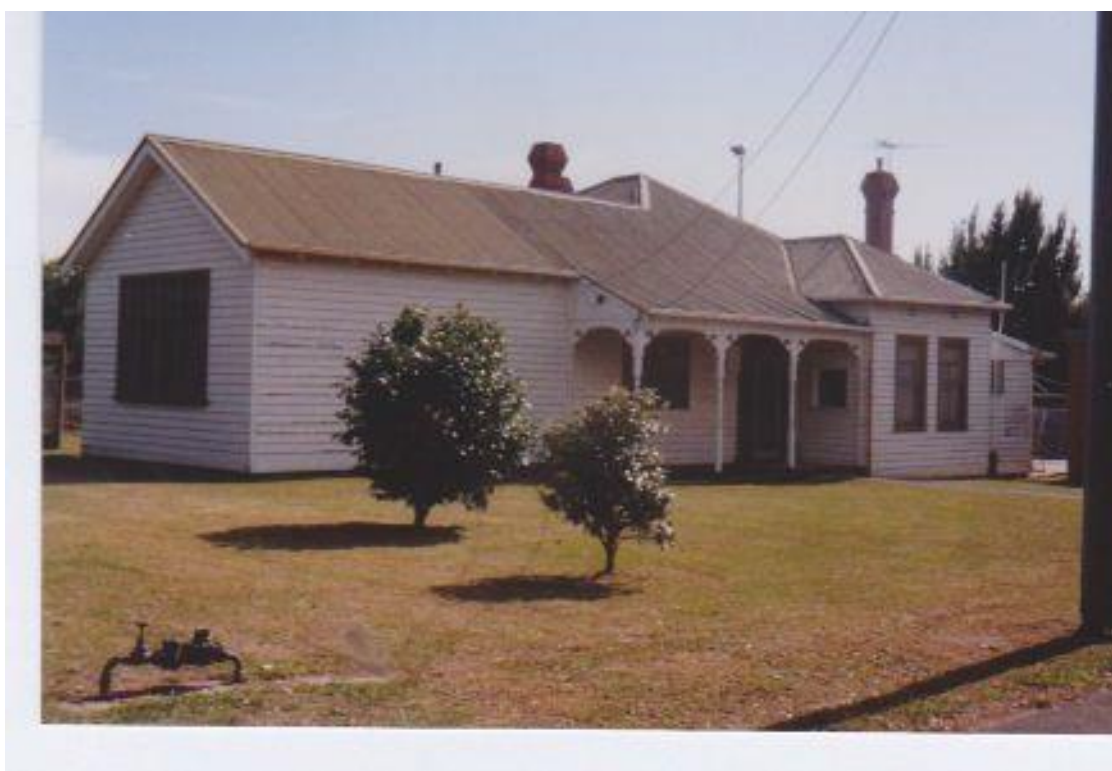
The original presbytery, an old farmhouse.
